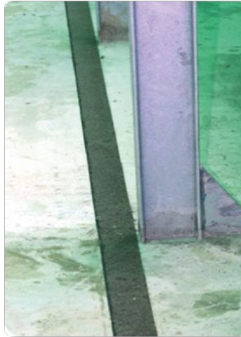
Figure 8 – Laying the bituminous strips
