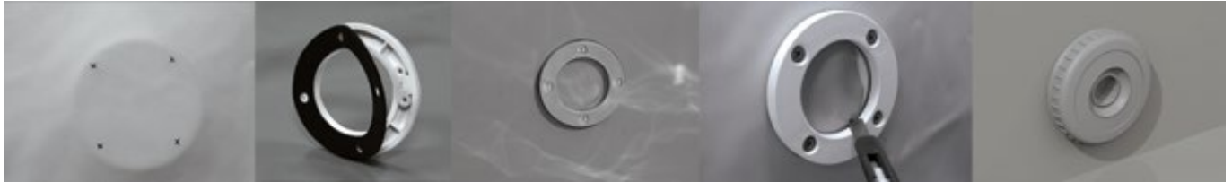
Figure 35 – Installing the return fitting flange
