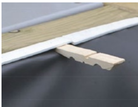
Figure 32 – Blocking the liner in position using half clothes pegs
