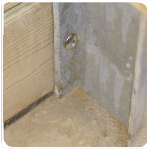
Figure 11 – Fastening the slats to the supporting braces
