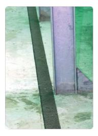
Figure 7 – Laying the bituminous strips
