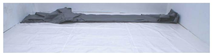
Figure 27 – Unfolding the liner
