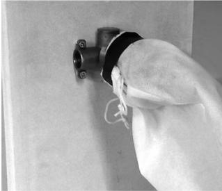
14. Next, cover the faucet to protect it while the wall is finished off. Make sure that no dust can reach the faucet.
