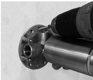
13. Affix the faucet to the structural rear wall using four screws, and connect the water supply as indicated.
